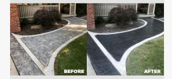
"The color in these pours were not integral. **Blasting removed the topical coloring along with the old sealer.** Used a medium gray for coloring, then antiqued it in black. The pads were then sealed with Deco Guard 25% high gloss sealer. The finished photos give the appearance that it's very dark, however in person it has a dark slate appearance." **Tri-City Blasting and Sealing**, Tri-City Area, MI
