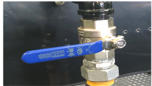
Figure 7. Valve is pictured in the closed position
